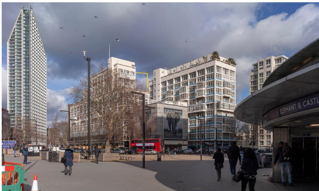
Image 52 (above): View from outside Elephant and Castle underground station entrance, looking northeast towards Metro Central Heights, with the outline of the proposed development indicated by the yellow line.
