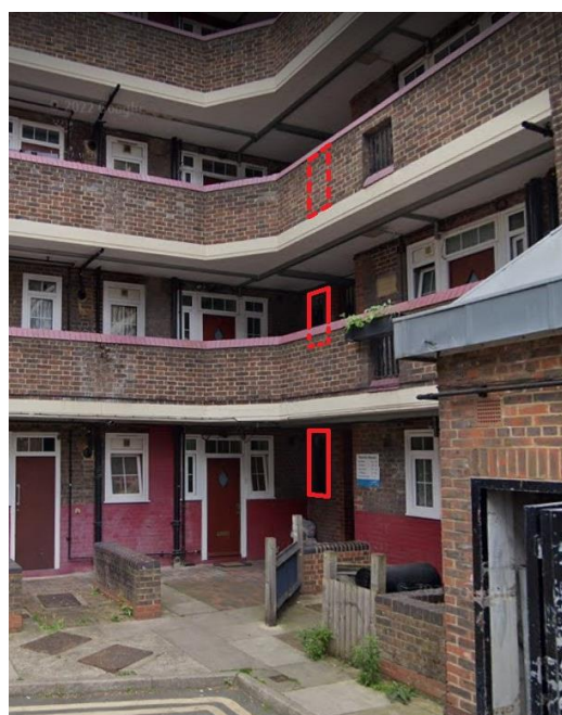
Image 41 (above): Photo of Rennie House, overlaid with the outlines of three of the five bedroom windows that would experience substantial adverse VSC percentage losses.
